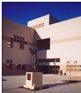
State Records Center and Archives Building located in Santa Fe
